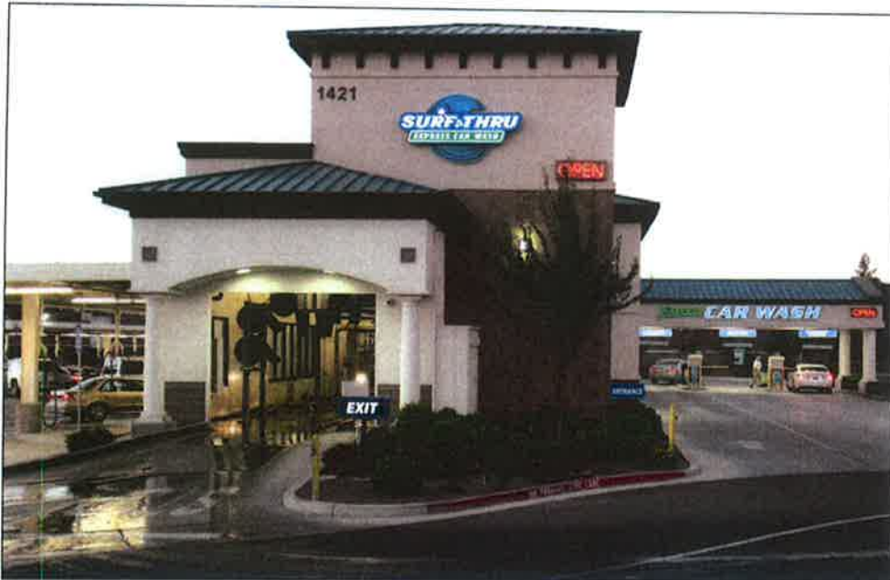
Photo 5 – Front Building Elevation
