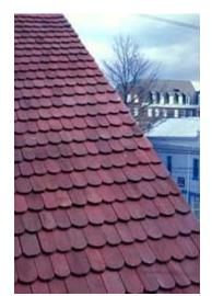
New rounded butt sawn shingles, with a smooth finish and red oxide stain, were used to replace the deteriorated shingles. The varying widths, between 4" and 7" will keep them from curling and cupping. Exposure length was determined from historic nail patterns on the historic spaced sheathing below. Photo: NPS files..
