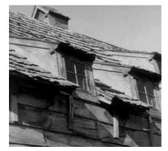
The long, biaxially tapered handsplit shingles are overlapped both vertically and horizontally. Photo: NPS files.
