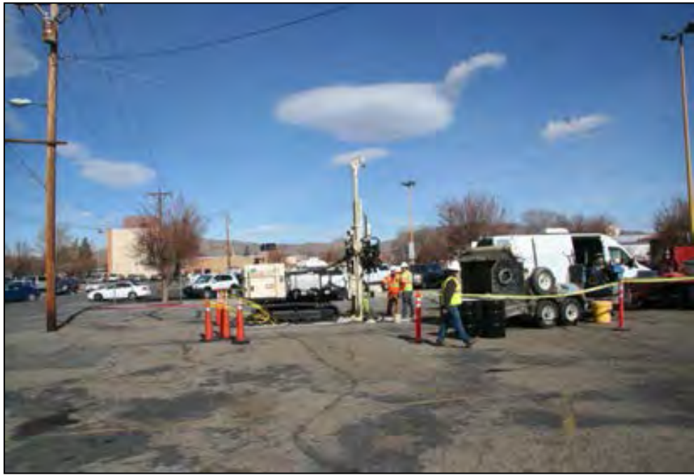
Photograph #3 Cone Penetration Test 1 Between Building B and Building C.
