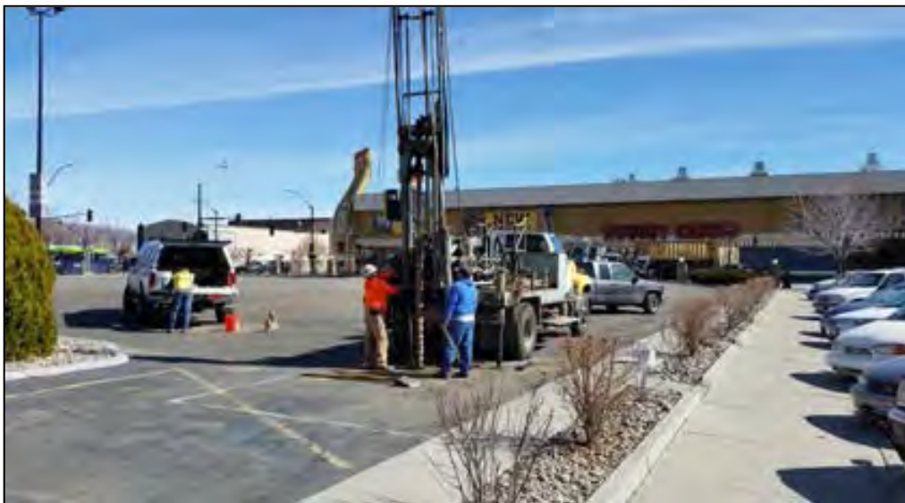
Photograph #2 Boring BH-9 Andresen Drilling SW Corner of Building A.
