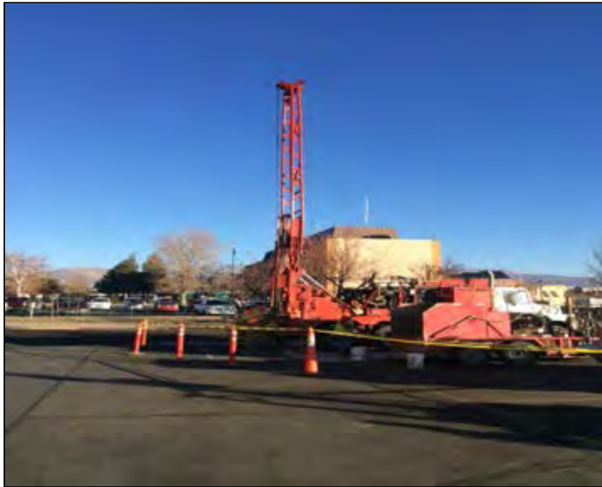
Photograph #1 Boring BH-2 Cascade Drilling NE Corner of Building B.
