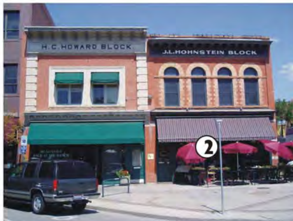
② Upper story doors and windows and street-level storefronts that have been previously covered, sealed, or filled in should be restored to their original proportions during the rehabilitation process.
