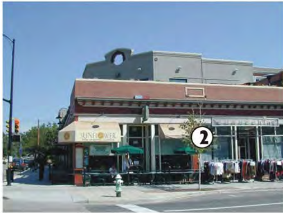
2 Display windows provide transparency at the street level of these retail storefronts, creating an inviting environment for pedestrians.
