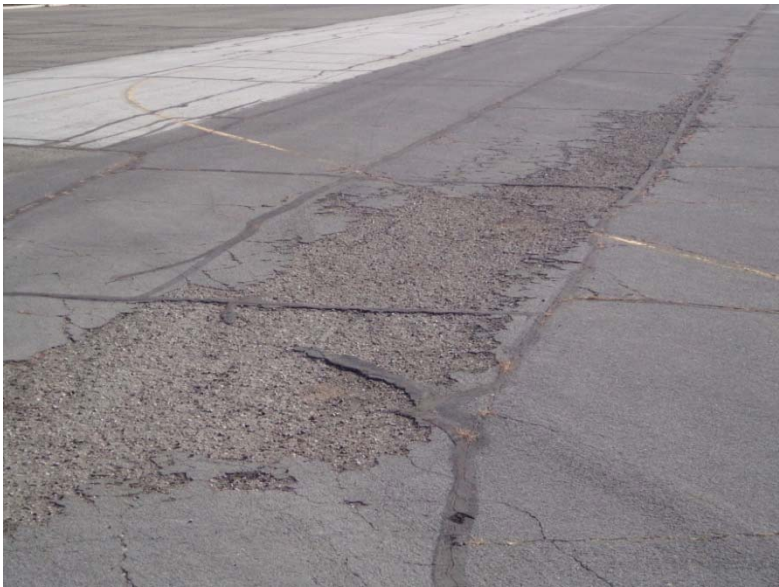
Typical raveling near the main taxilane in the north apron
