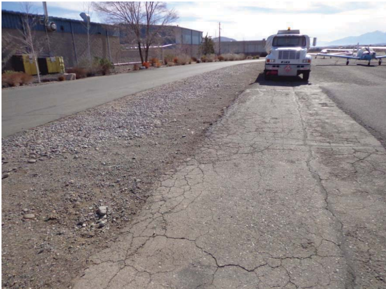
Typical edge of apron pavement at the apron access road
