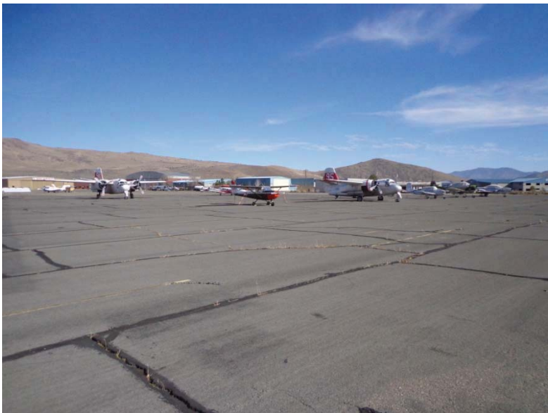
North Apron looking north from the perimeter road
