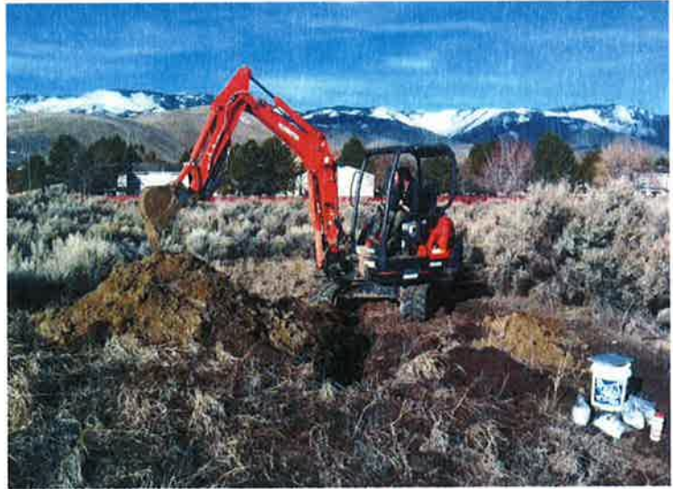
Test Pit Exploration
