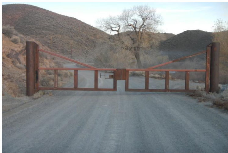
Existing swing gate Brunswick Canyon Road heading east into Carson River Canyon
