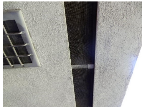
Juvenile Detention Soffit Vents
