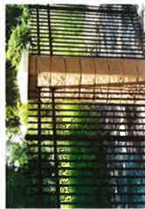
8 FT. METAL FENCE WITH PILLARS
