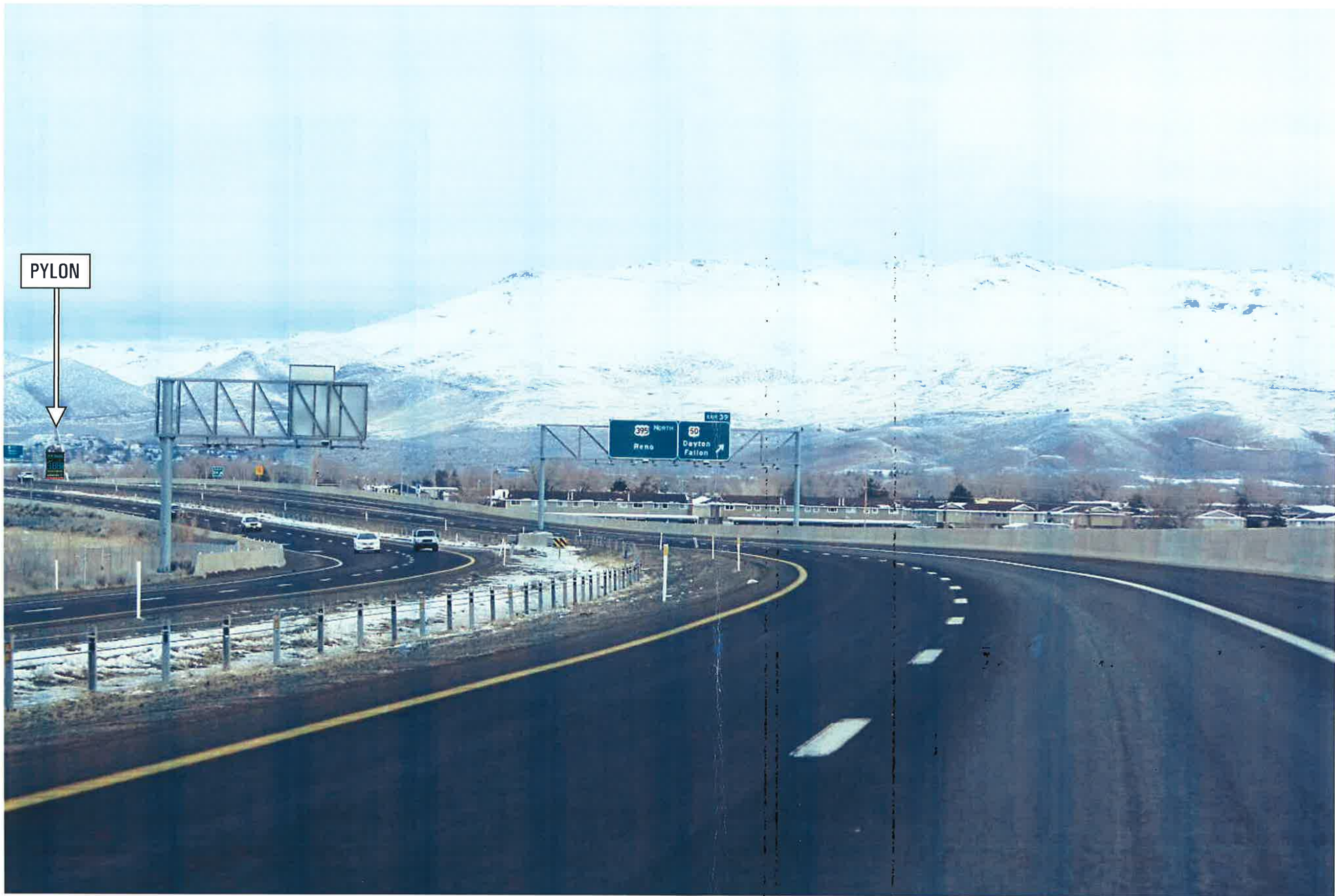
NORTHBOUND FREEWAY - FAR PYLON @ 47'-7" HEIGHT
