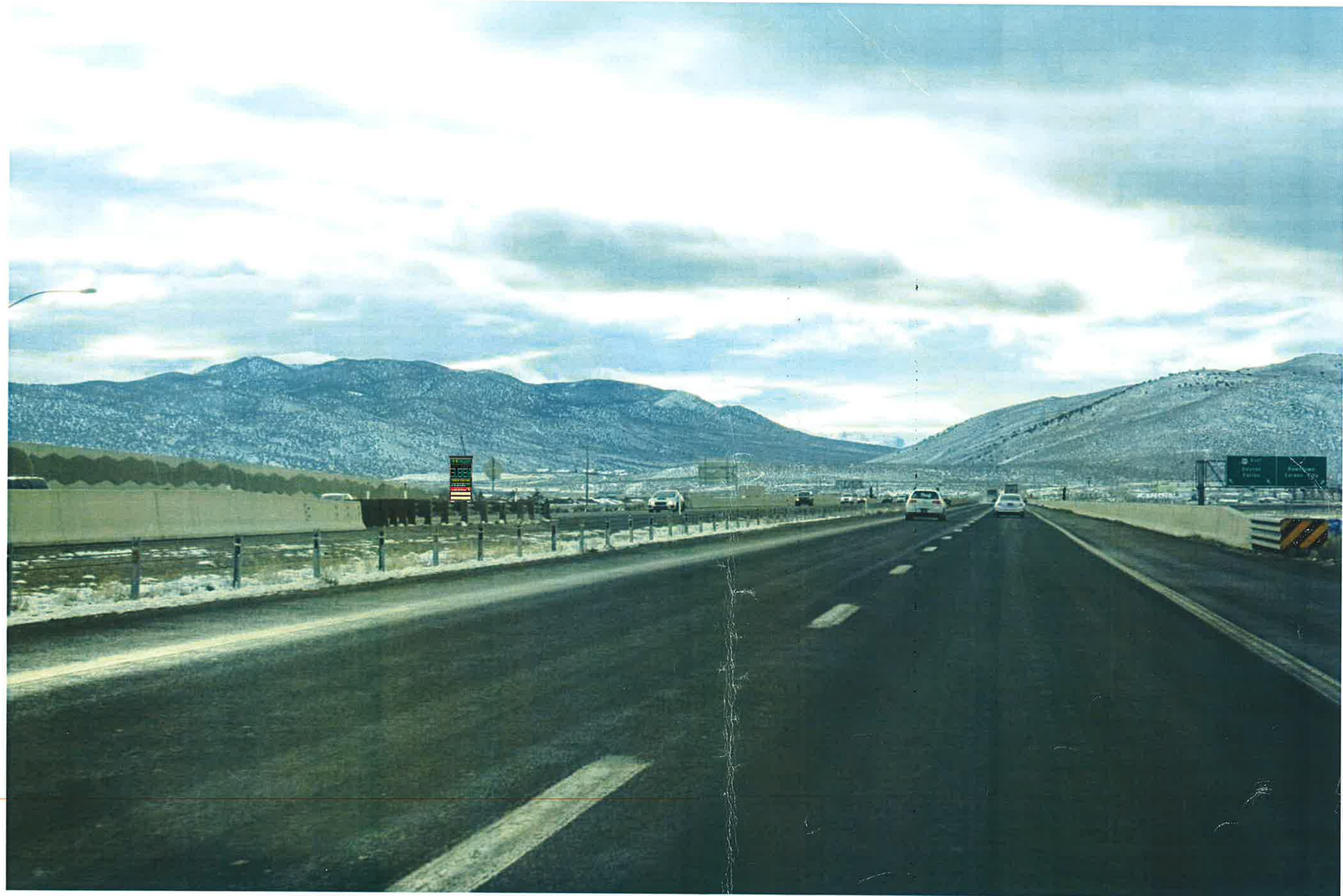
SOUTHBOUND FREEWAY - MID
