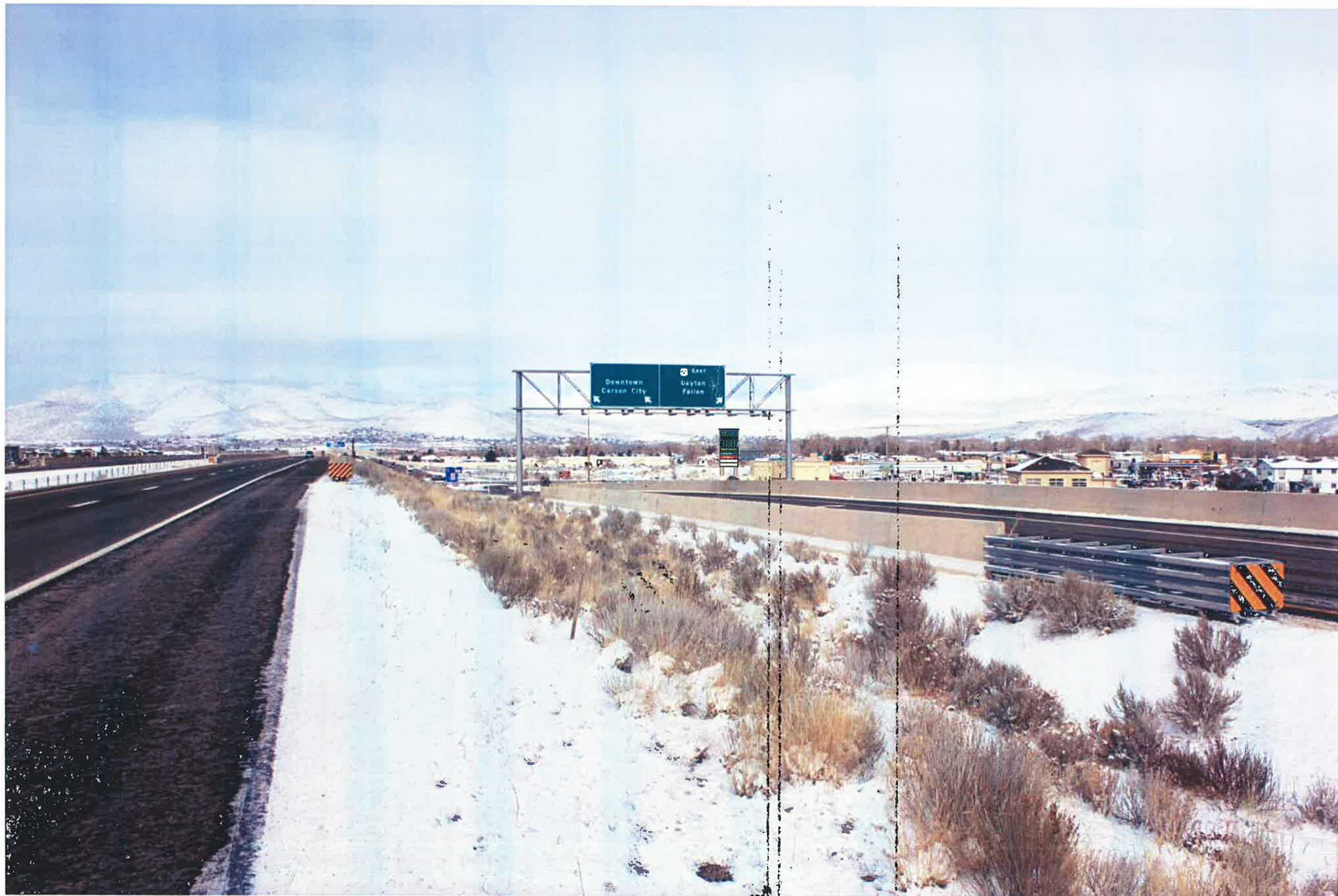
NORTHBOUND FREEWAY - 1,000 FEET PYLON @ 47'-7" HEIGHT
