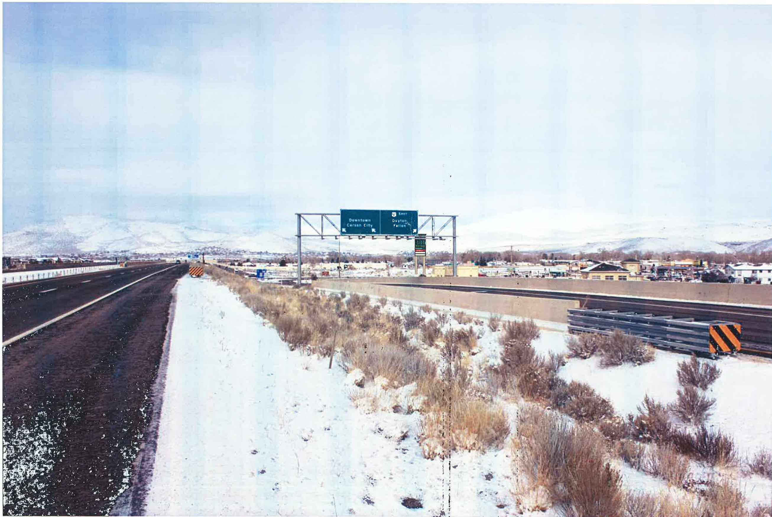
NORTHBOUND FREEWAY - 1,000 FEET PYLON @ 67'-7" HEIGHT
