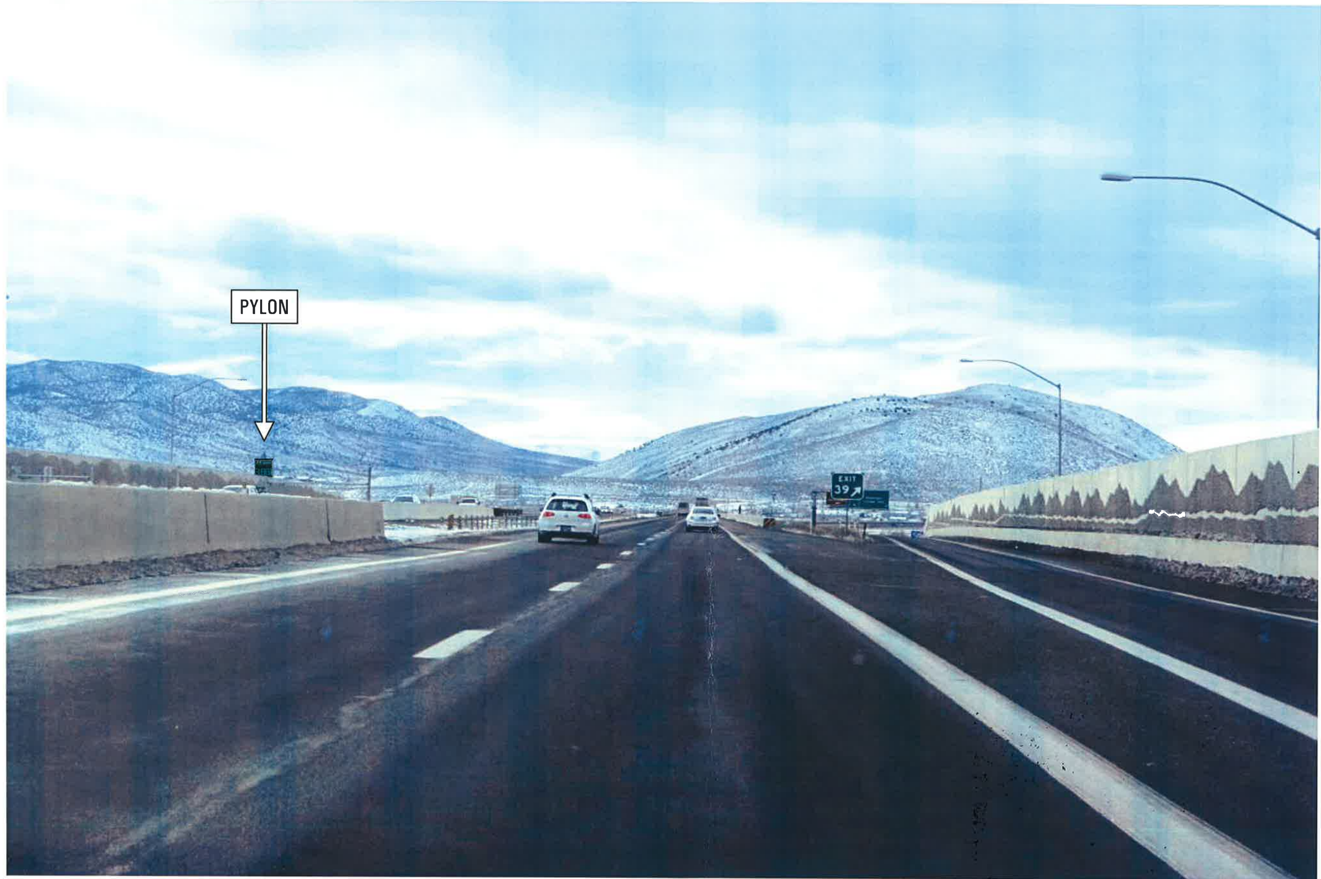
SOUTHBOUND FREEWAY - FAR PYLON @ 67'-7" HEIGHT
