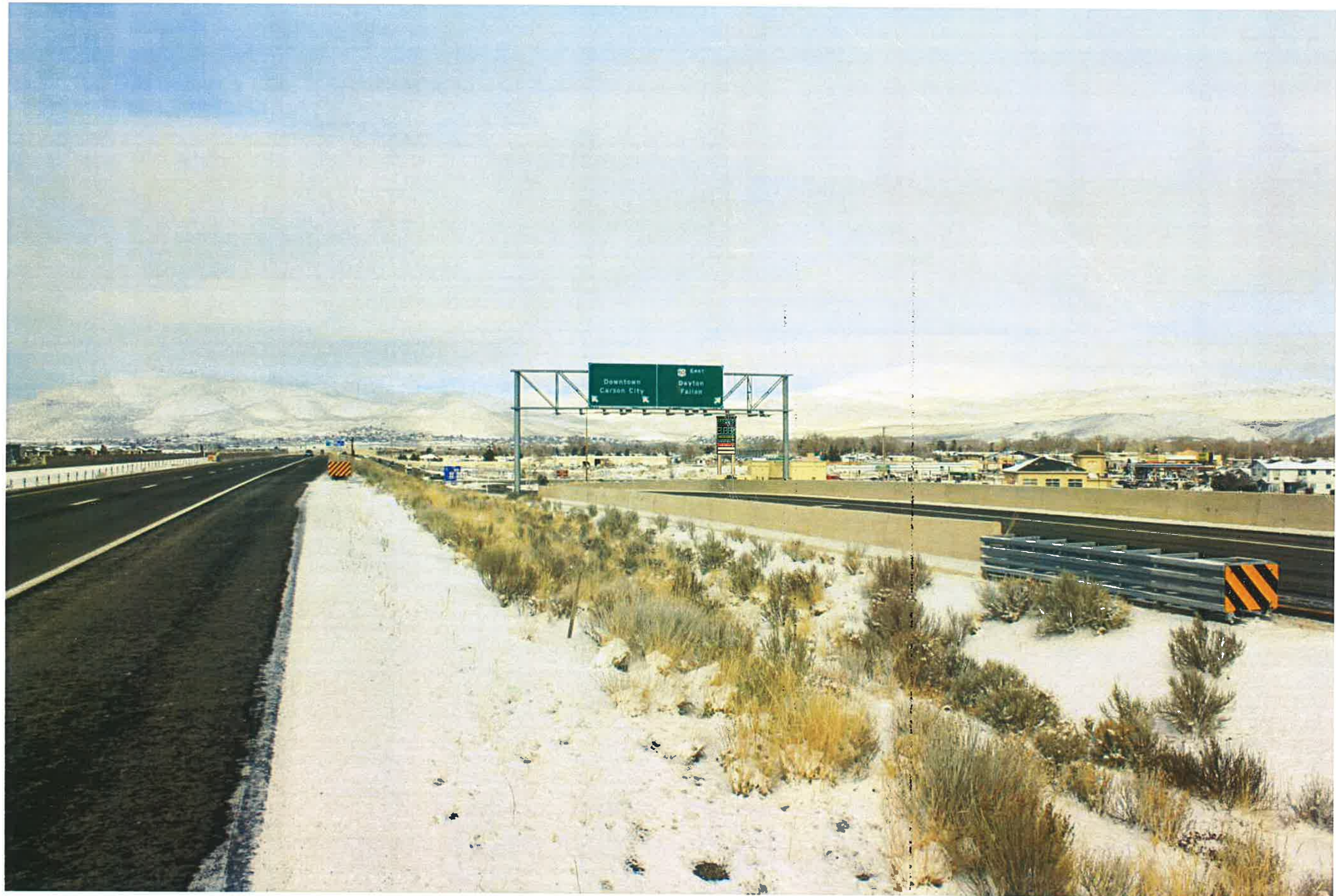
NORTHBOUND FREEWAY - 1,000 FEET
