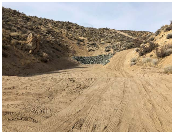
Golden Eagle Lane Erosion Control Project – newly constructed detention basin and culvert.
