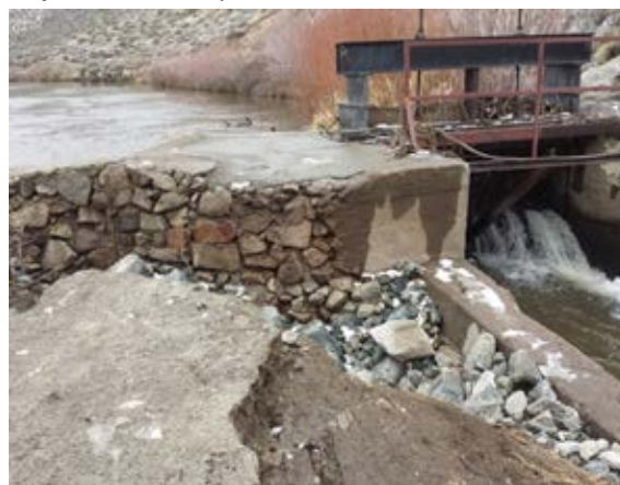
Mexican Dam – flood damage from January 2017
