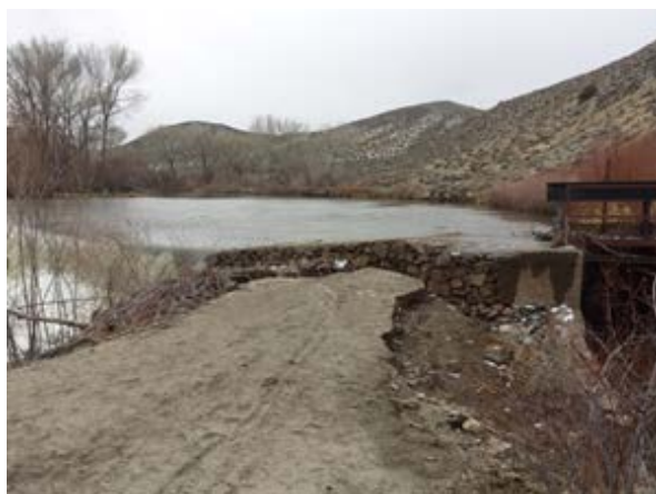
Mexican Dam – flood damage from January 2017
