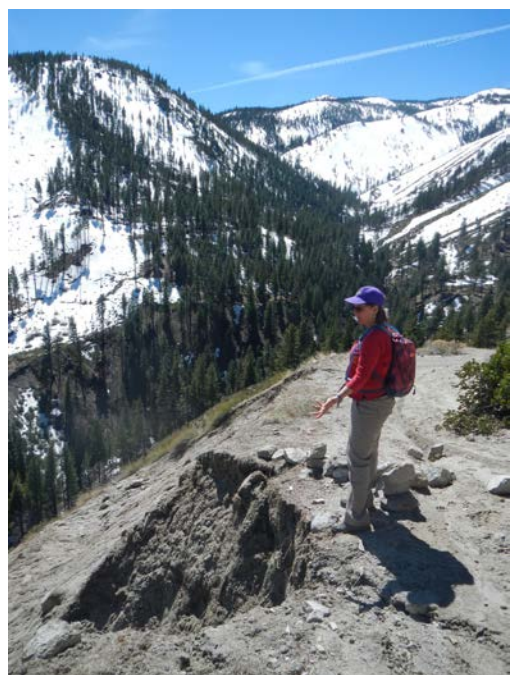
Ash Canyon road damage from 2017 storm events
