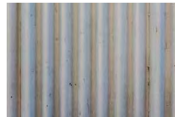
Corrugated metal roofs for sign kiosks
