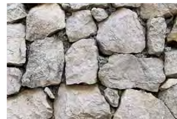
Dry or wet-stacked stone walls
