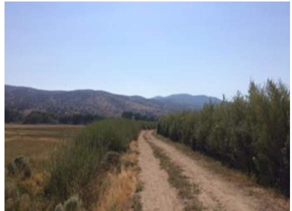
After: pruning and removing willows along the road/trail.
