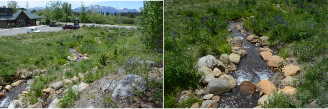
Burke Creek Post Construction June 2018
