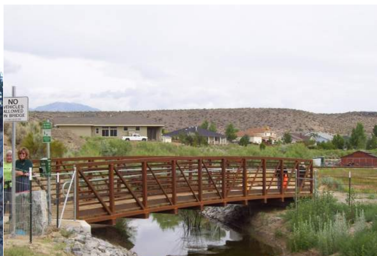
Existing Bridge over the Mexican Ditch
