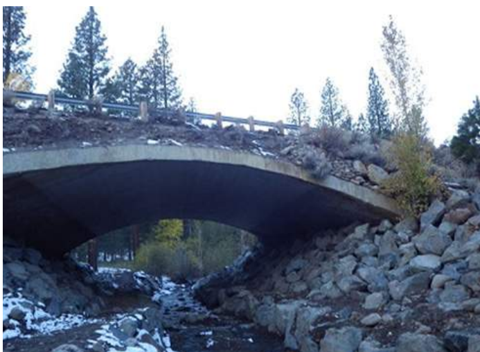
Galena Creek Trail at Joy Lake Road Bridge
