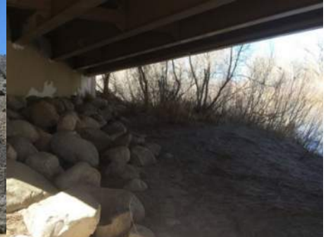
Under the Carson River Road Bridge
