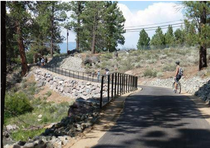
Truckee River Legacy Trail Phase 3B – Alignment fits terrain on steep side-slope
