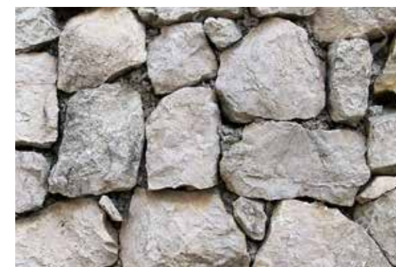
Dry or wet-stacked stone walls
