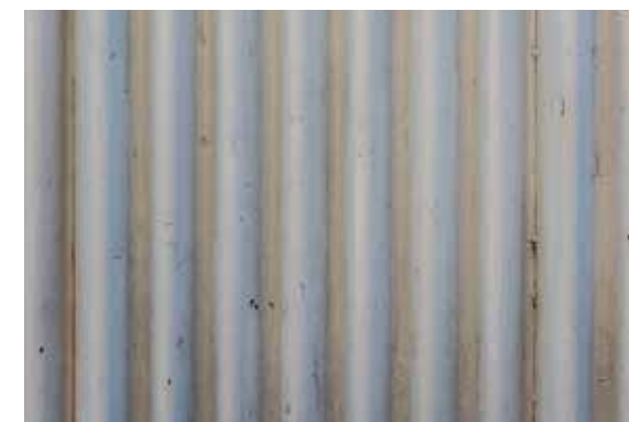
Corrugated metal roofs for sign kiosks
