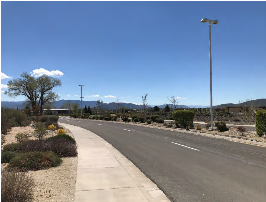
Photograph 12: View of the southern Property boundary and southern adjoining property.
