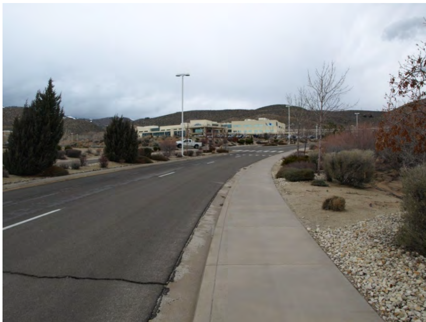
VIEW LOOKING NORTHWEST ON MEDICAL PARKWAY FROM NEAR THE SOUTHWEST CORNER OF THE SUBJECT
