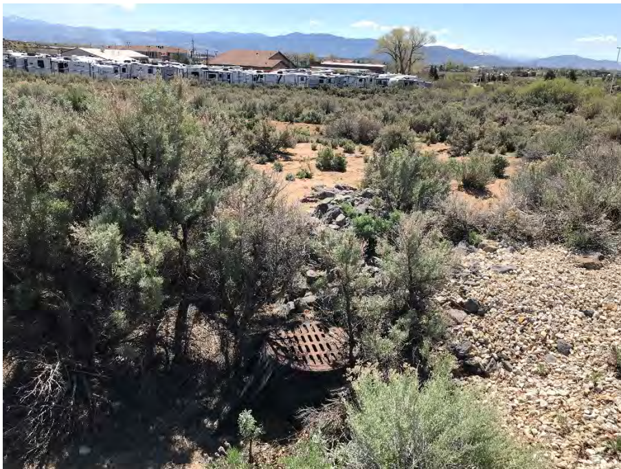
Photograph 4: View of a catch basin near the western Property boundary.
