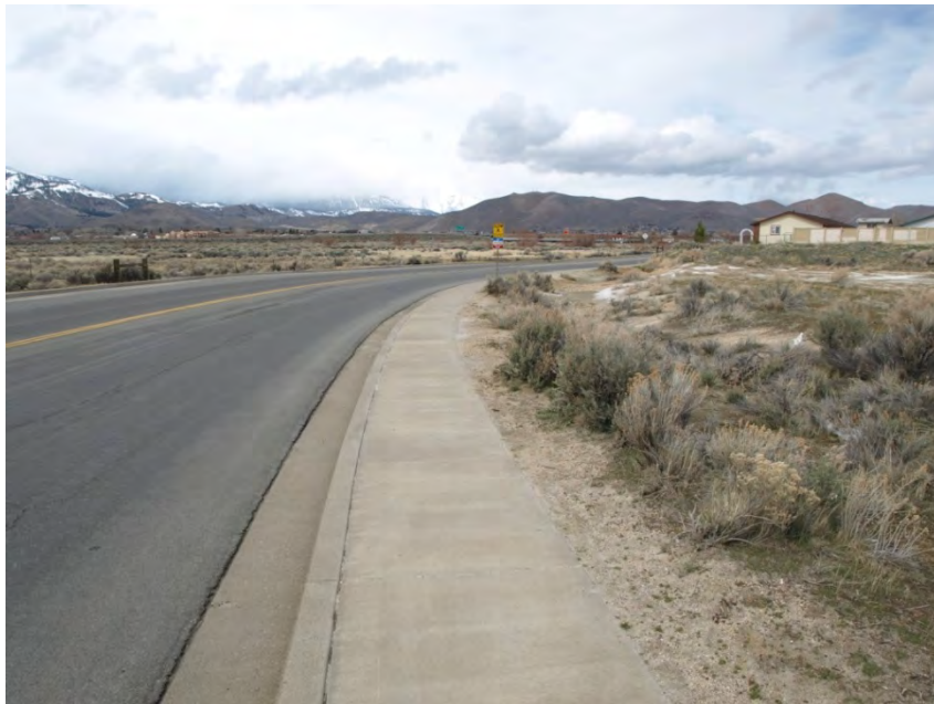
VIEW LOOKING NORTHWEST ON AIRPORT ROAD FROM NEAR THE SOUTHWEST CORNER OF THE SUBJECT
