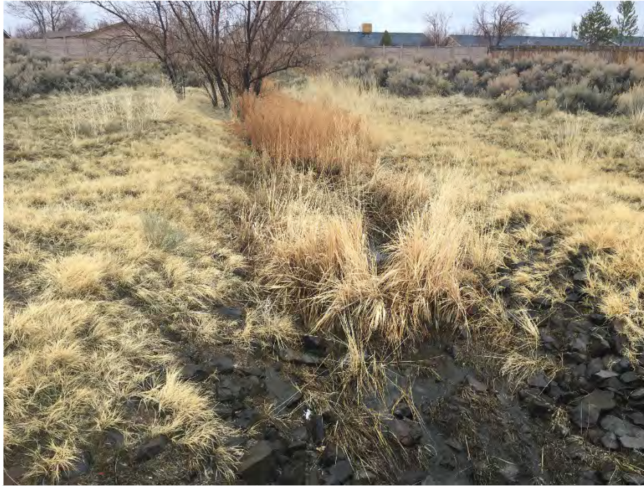
Picture 13: Drainage channel in central portion of Property.
