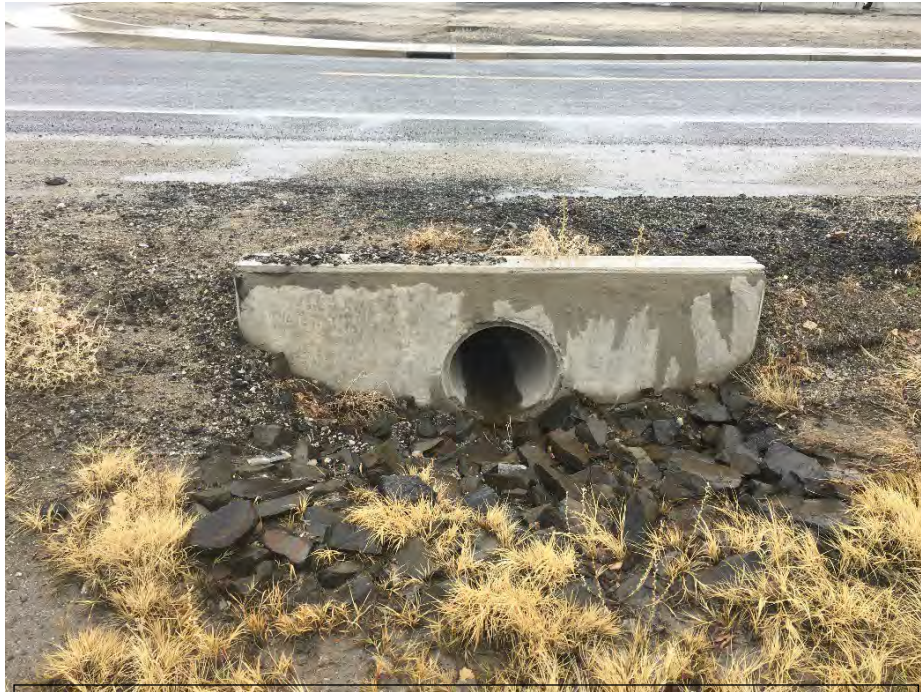
Picture 11: Drainage ditch running under Butti Way north to south in central portion of the Property.
