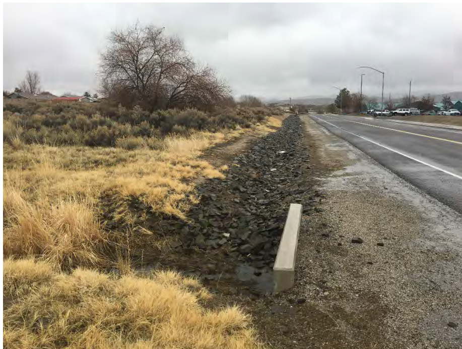
Picture 12: Drainage ditch running along Butti Way north to south in central portion of the Property.
