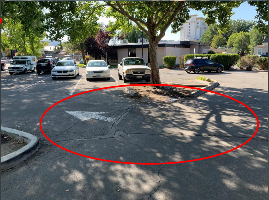
Tree Roots Damaging Infrastructure
