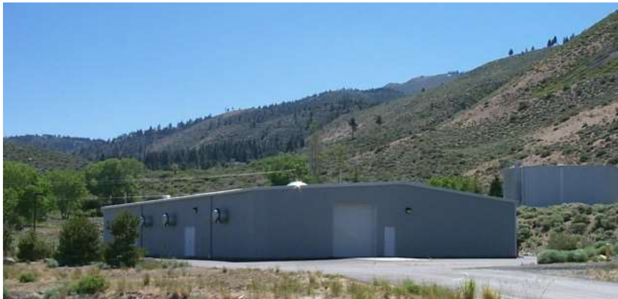
Quill Water Treatment Plant
