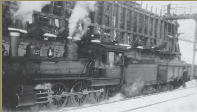
V & T locomotive #25 delivering building materials to the mill during construction. Joe Curtis Collection.
