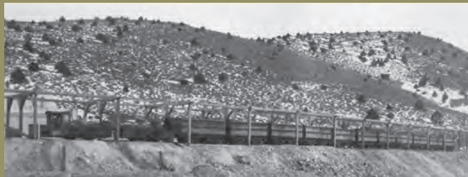
An ore train, with its electric battery locomotive, brought ore from the workings in Gold Hill and Virginia City to Building 1, the Ore Bin. Joe Curtis Collection.
