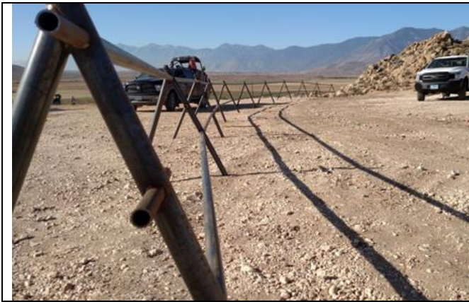
Jack Rail fencing installed to identify boundaries and restricted areas.
