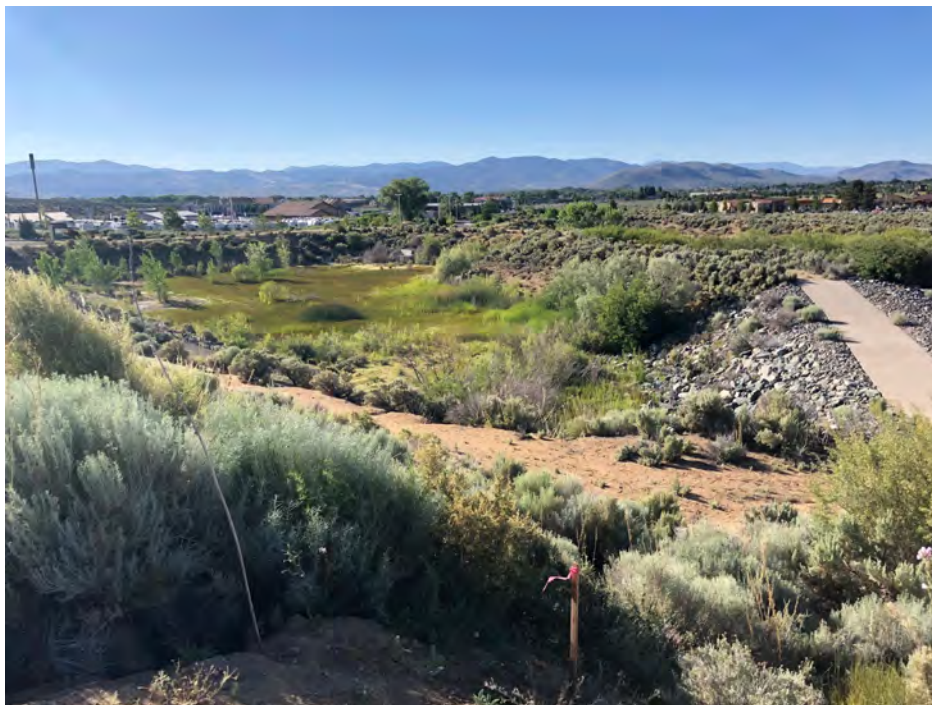
Photo 3. Site conditions in created detention basin #1 in July, 2019.
