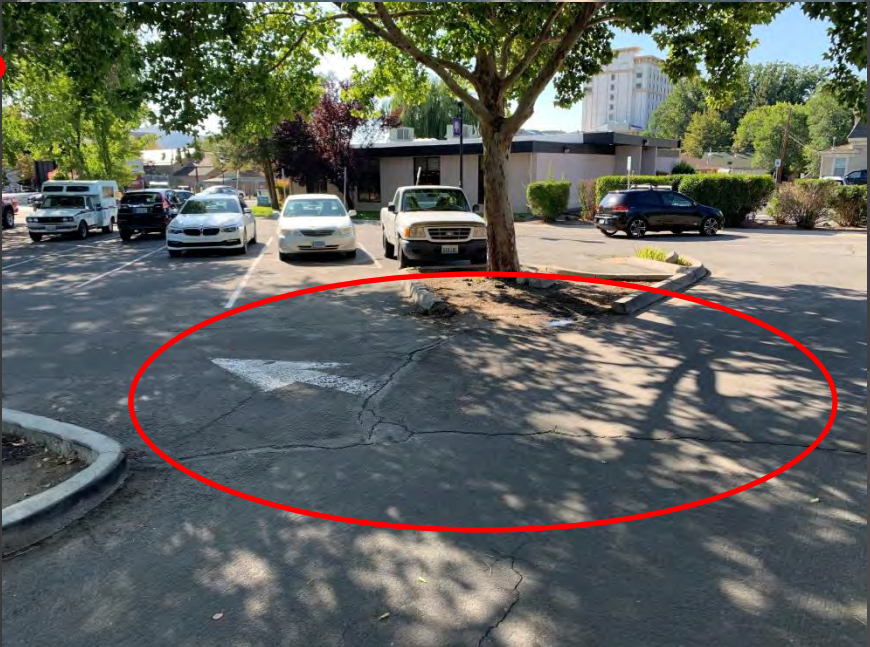
Tree Roots Damaging Infrastructure
