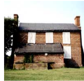
Appropriately mothballed historic building. Photo: NPS files.
