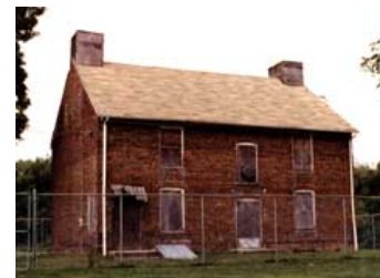
A view showing the exterior of the Brearley House, New Jersey, in its mothballed condition. Photo: Michael Mills, Ford Farewell Mills Gatsch, Architects.
