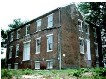
This building has been successfully mothballed for 10 years because the roof and walls were repaired and structurally stabilized, ventilation louvers added, and the property maintained. Photo: NPS files.
