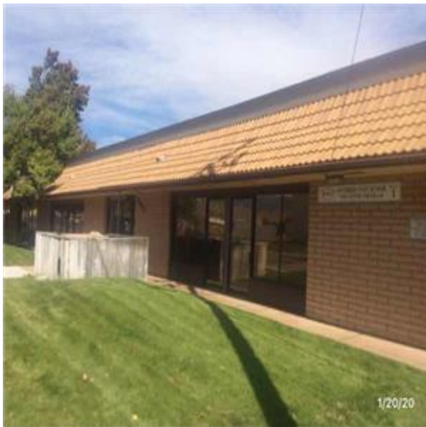
View of Clay Roof Tile
