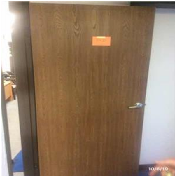
View of Interior Single Wood Door(s)
