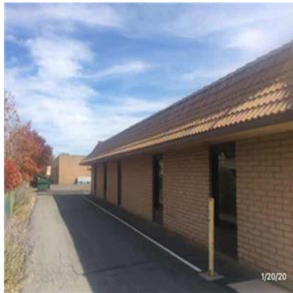
B3016 Gutters and Downspouts :- View of Aluminum Perimeter Gutters
