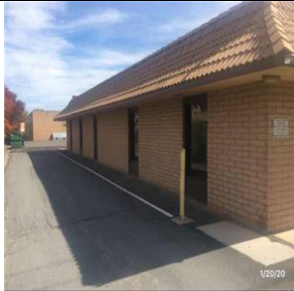
B2011 Exterior Wall Construction :- View of Veneer Brick
