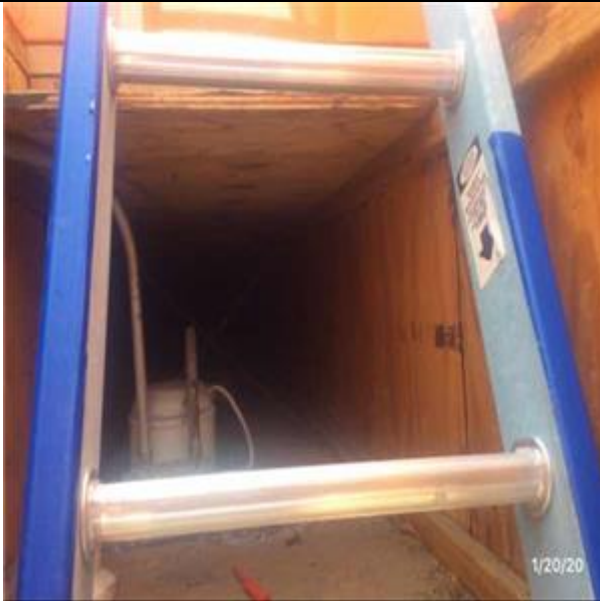
View of Wood Joists Supporting Exterior Grade Plywood
