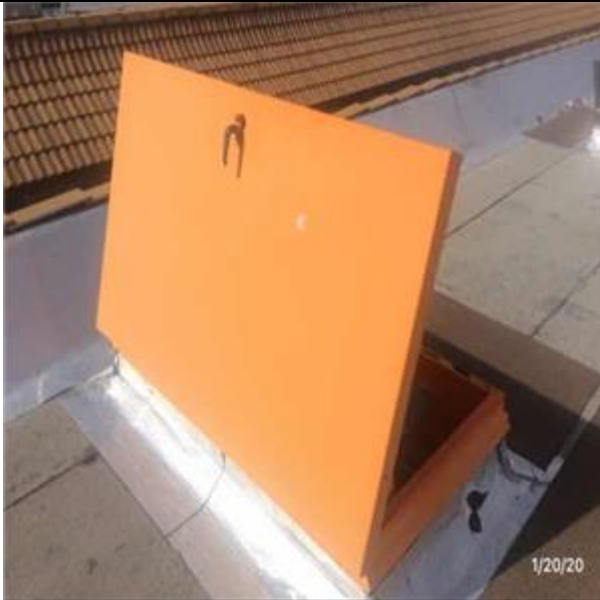
View of Galvanized Steel Hatch
