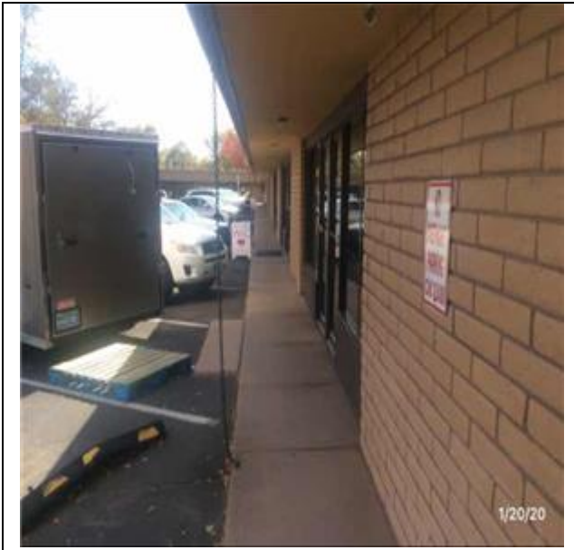
View of Concrete 3' - 4' Wide
