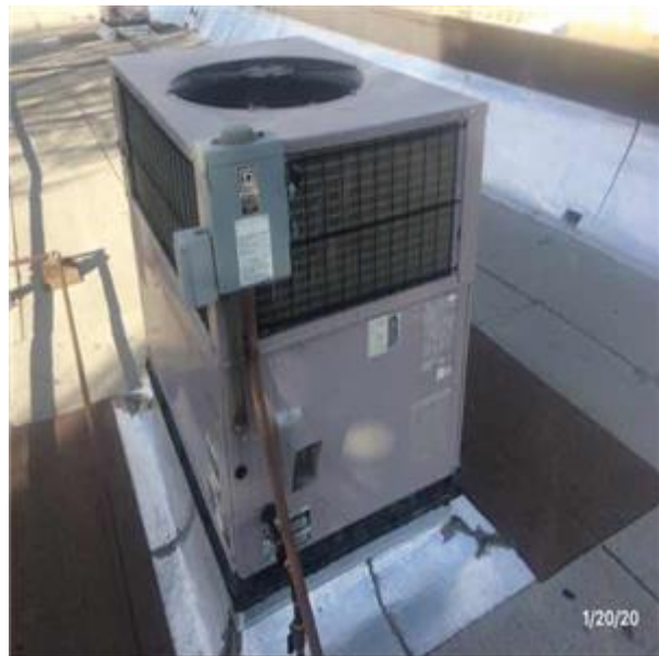
D3052 Package Units :- View of Packaged Rooftop A/C With Heat, Under 20 Tons - E-3
