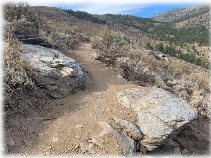
A completed segment of Lincoln Bypass
