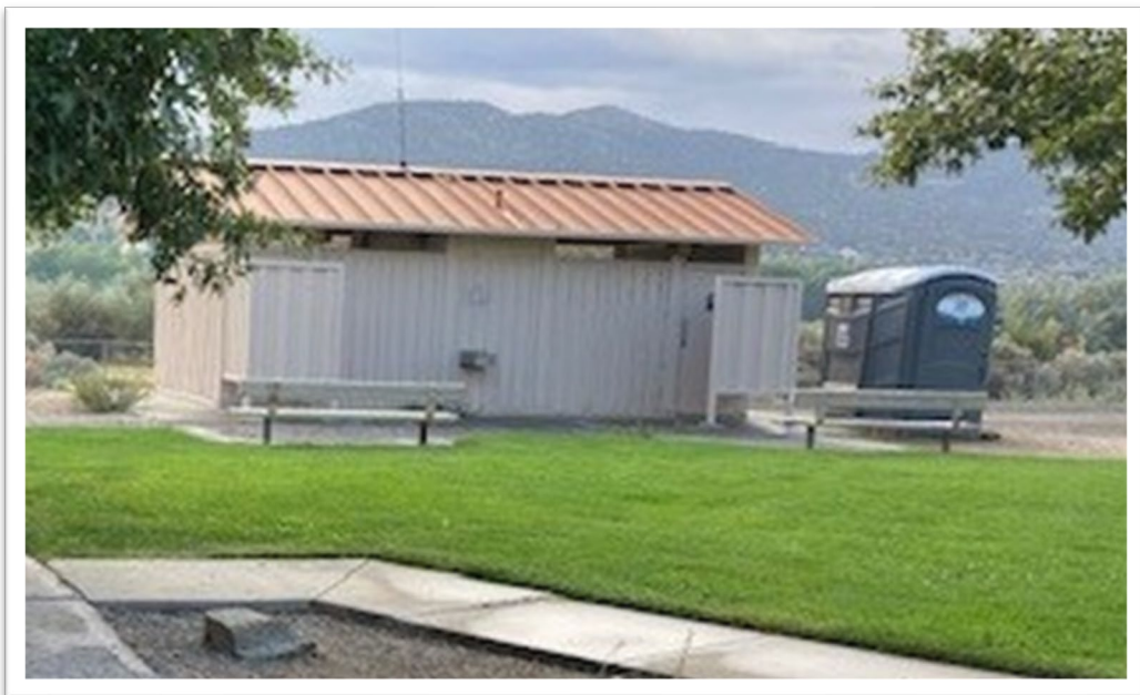
Existing toilet to be replaced.
