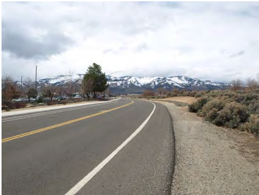
VIEW LOOKING WEST ON BUTTI WAY FROM NEAR THE SOUTHEAST CORNER OF THE SUBJECT'S LARGER PARCEL
