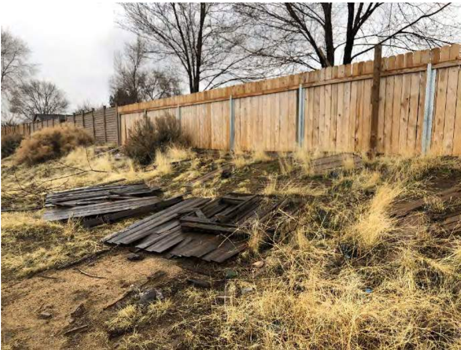
Picture 20: Remains of wooden fencing next to new fencing on northern central portion of Property.
