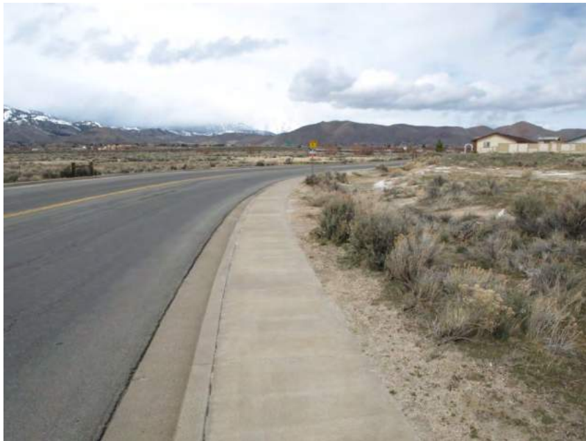
VIEW LOOKING NORTHWEST ON AIRPORT ROAD FROM NEAR THE SOUTHWEST CORNER OF THE SUBJECT
