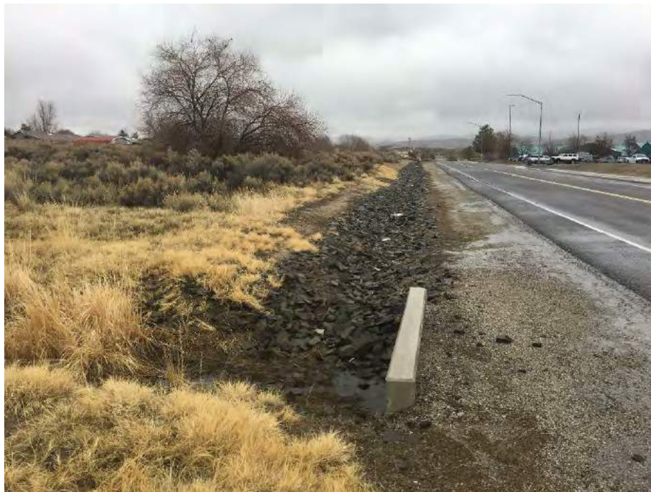
Picture 12: Drainage ditch running along Butti Way north to south in central portion of the Property.
