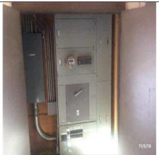
D5012 Low Tension Service & Dist :-View of Switchboard - 120/208volts, 400 to 2000amp
