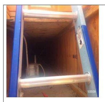
View of Wood Joists Supporting Exterior Grade Plywood
