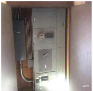
D5012 Low Tension Service & Dist :-View of Switchboard - 120/208volts, 400 to 2000amp
