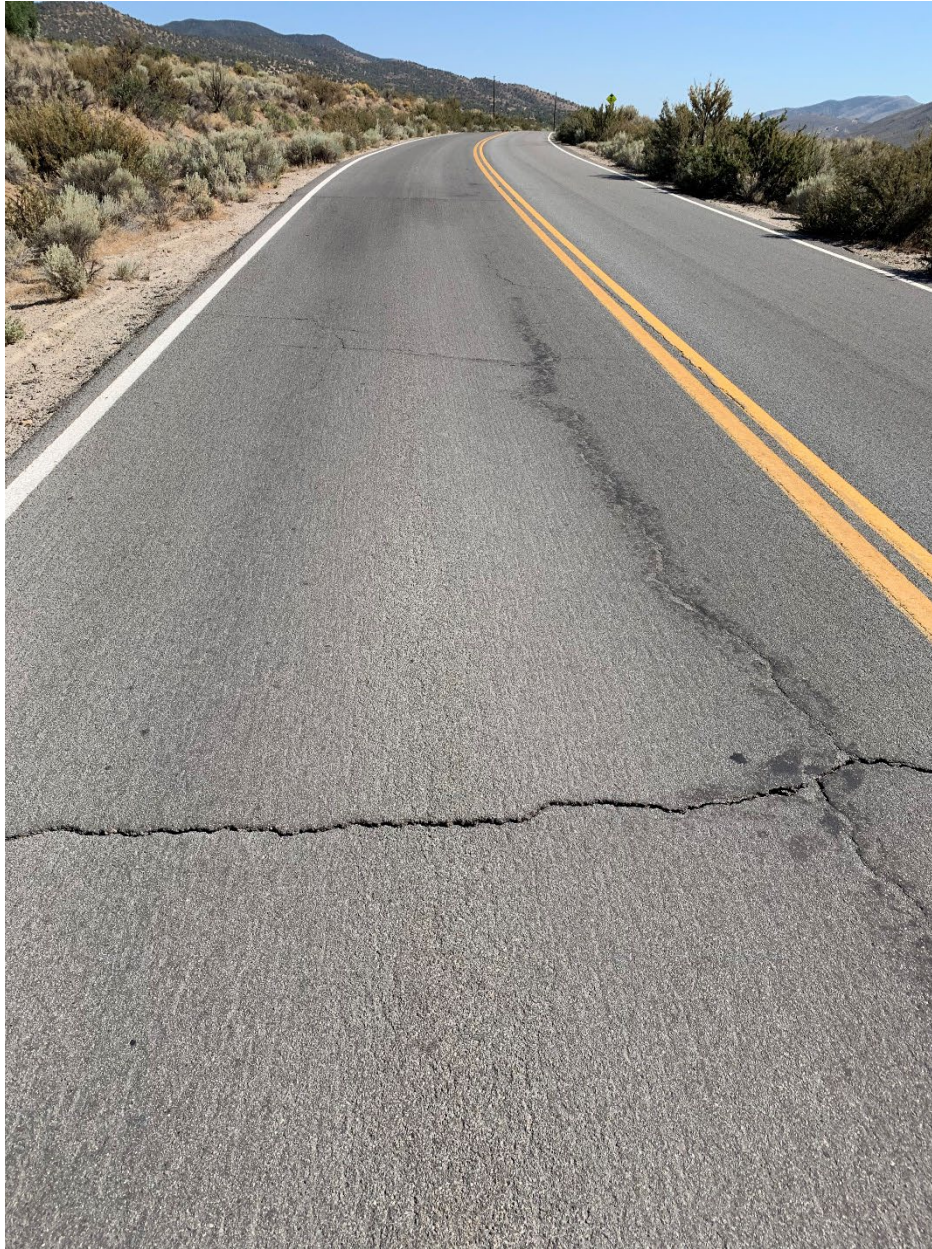
Figure 4. Pavement in Fair condition category (PCI 70-56).
