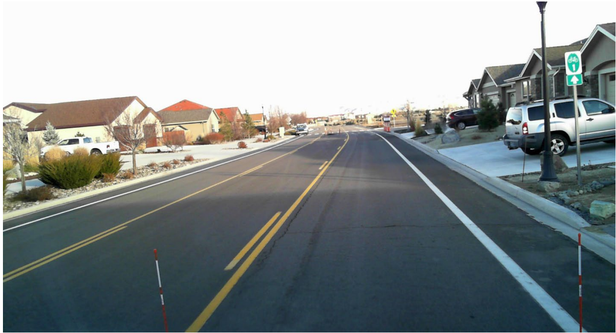
Figure 3. Pavement in Satisfactory condition category (PCI 85-71).
