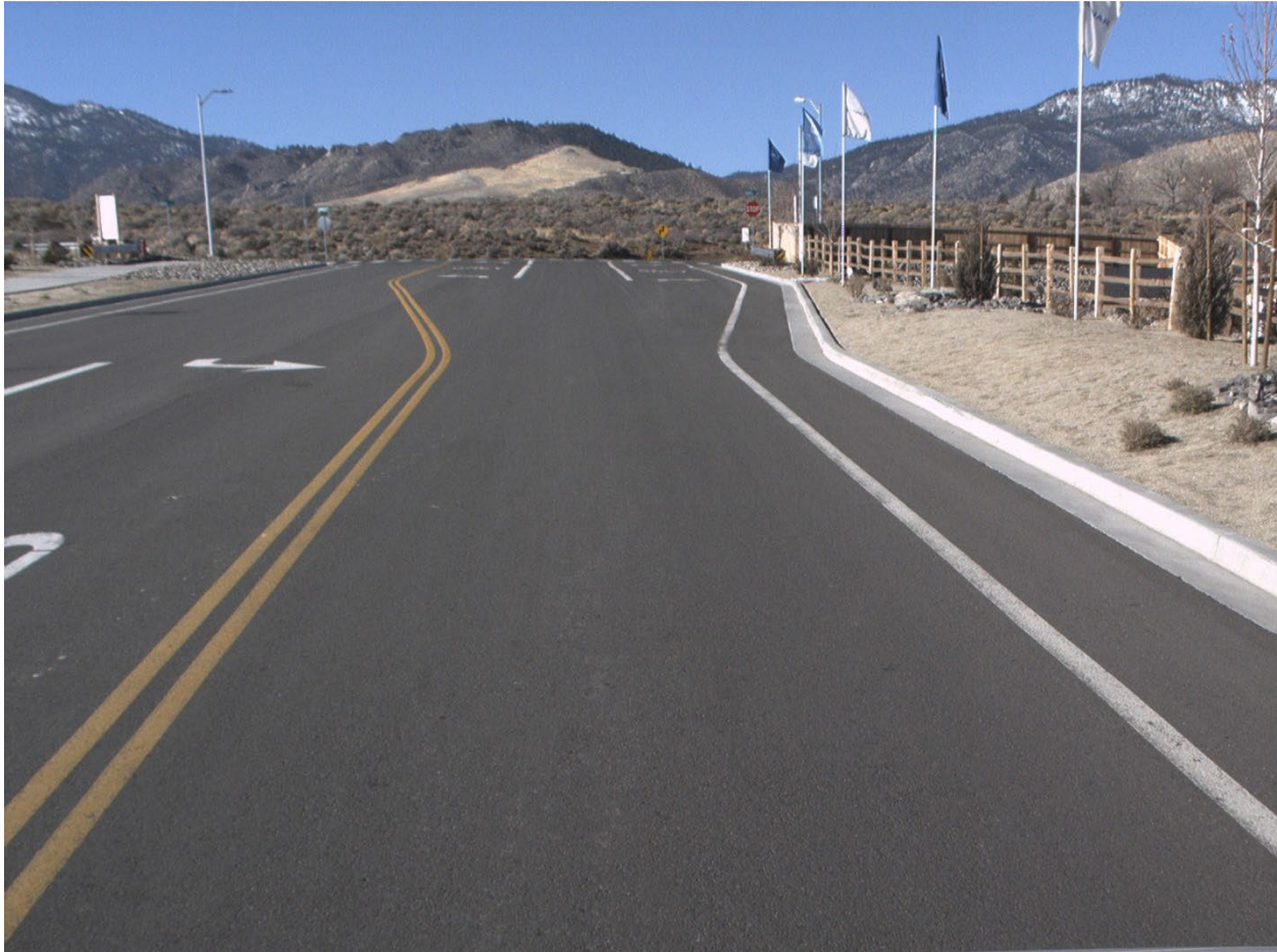
Figure 2. Pavement in Good condition category (PCI 100-86).
