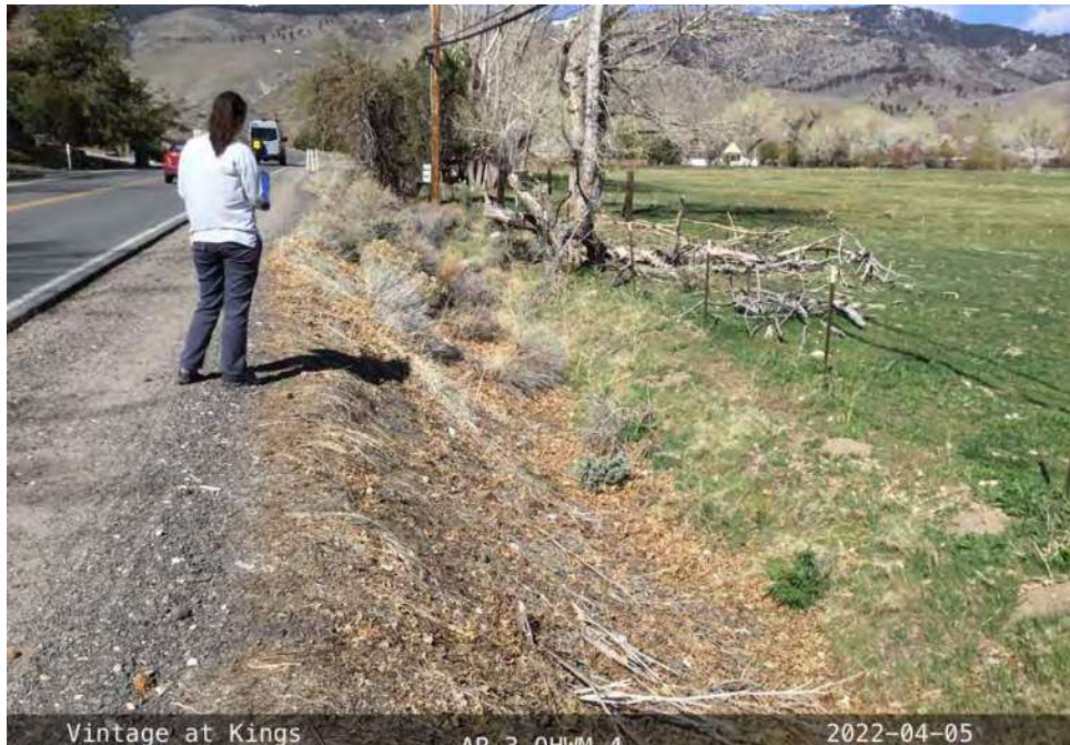
Photo 9. OHWM-4: AR-3 excavated roadside ditch at eastern end when some overland flow from irrigated pasture may intermittently be entering ditch. View looking west.
