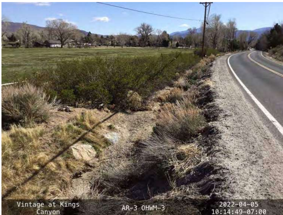
Photo 8. OHWM-3: AR-3 excavated roadside ditch capturing storm water from road. When present, water flow from west to east into storm drain at southeast corner of Survey Area. View looking east.
