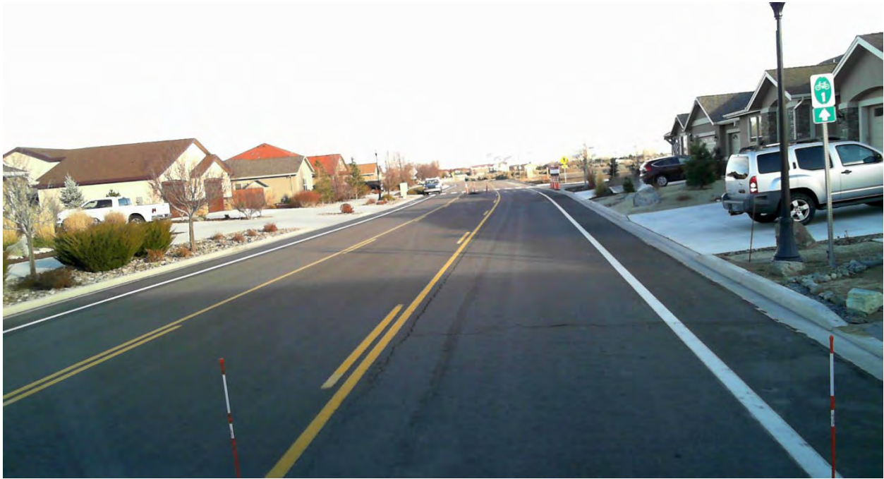
Figure 3. Pavement in Satisfactory condition category (PCI 85-71).
