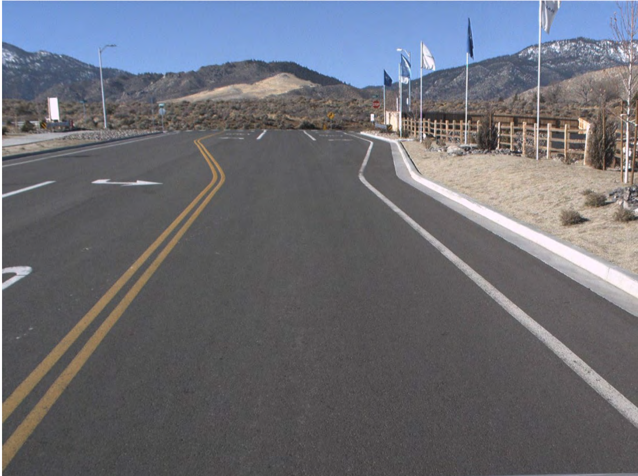
Figure 2. Pavement in Good condition category (PCI 100-86).
