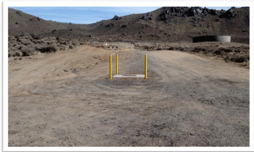
Photo 7. Koontz Lane below the water tank
