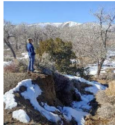
Laurel Road Headcut at Downstream Discharge
