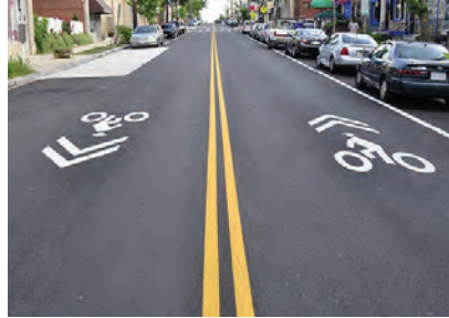
Sharrows also serve as positional guidance and raise bicycle awareness where there is not space to accommodate a full-width bike lane. Center lane markings may or may not be necessary depending on travel lane widths. Narrower two way residential streets (less than 22 ft between parked cars) have a natural traffic calming effect without center turn lanes.
