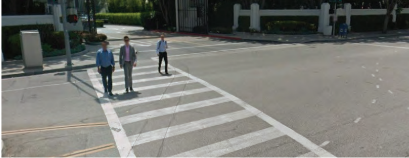
Marked crosswalks include standard parallel pavement markings as well as high-visibility ladder markings. Source: Google Streetview
