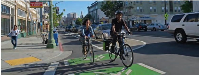
Parked cars serve as a barrier between bicyclists and the vehicle lane. Barriers could also include flexible posts, bollards, planters, or other design elements. Source: Bike East Bay
