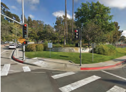
Not recommended: diagonal curb ramp configuration. Source: Google Streetview
