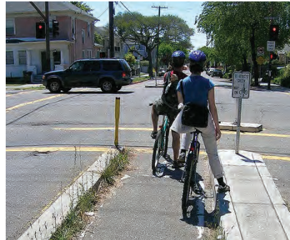
A bicycle detection system triggers a change in the traffic signal when a bicycle is detected.
