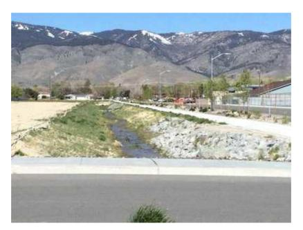
A special blend of vegetation has been planted along the drainage basins to prevent erosion and washout. Rockery rip rap and concrete culverts were constructed along the inlets in accordance with the Carson City Specs.
